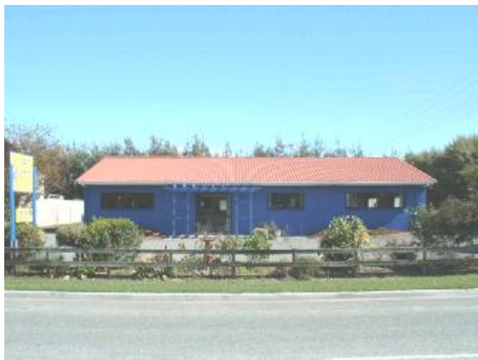
Building Progress to date
